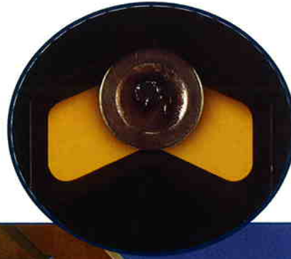
Detail view of pad and weld washer
