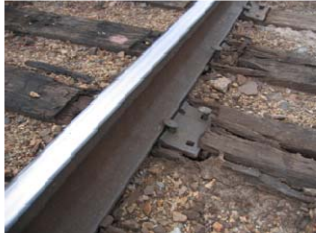
Figure 6. Broken screw spikes in a high-speed turnout.
