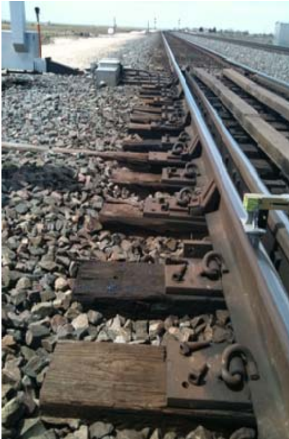
Figure 5. Spike-killed ties with plate cutting at a GWP exception.
